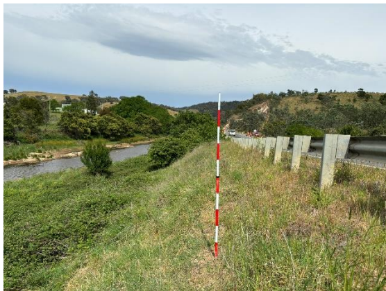
Plate 5: East extent of Project Area along south verge with view of Mulwaree River (West)
