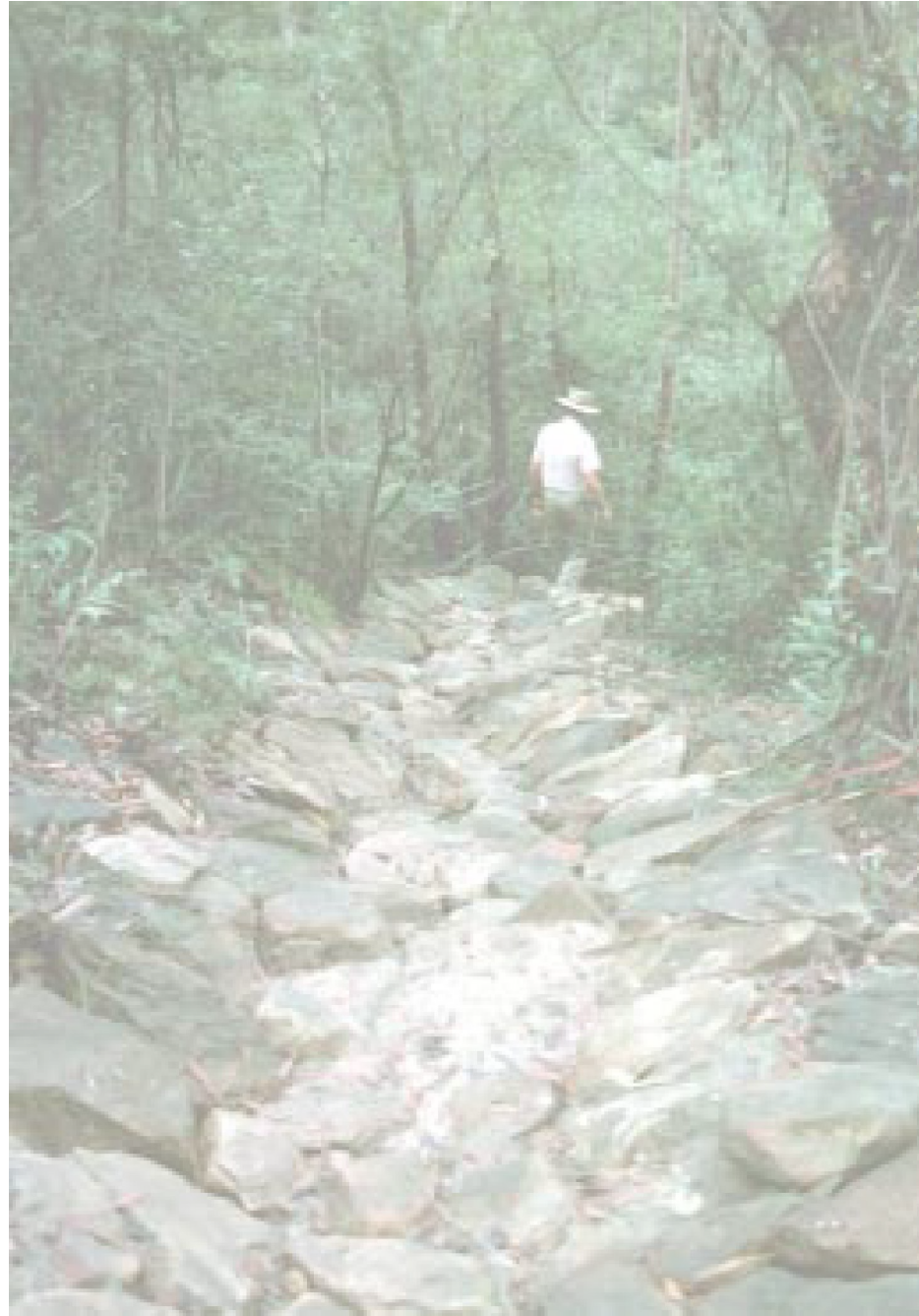
SOILS & CONSTRUCTION FIGURE 5.4 ROCK LINED WATERWAY
