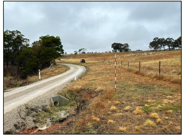
Plate 6. Western end of proposed material stockpile location and concrete culvert (southeast)
