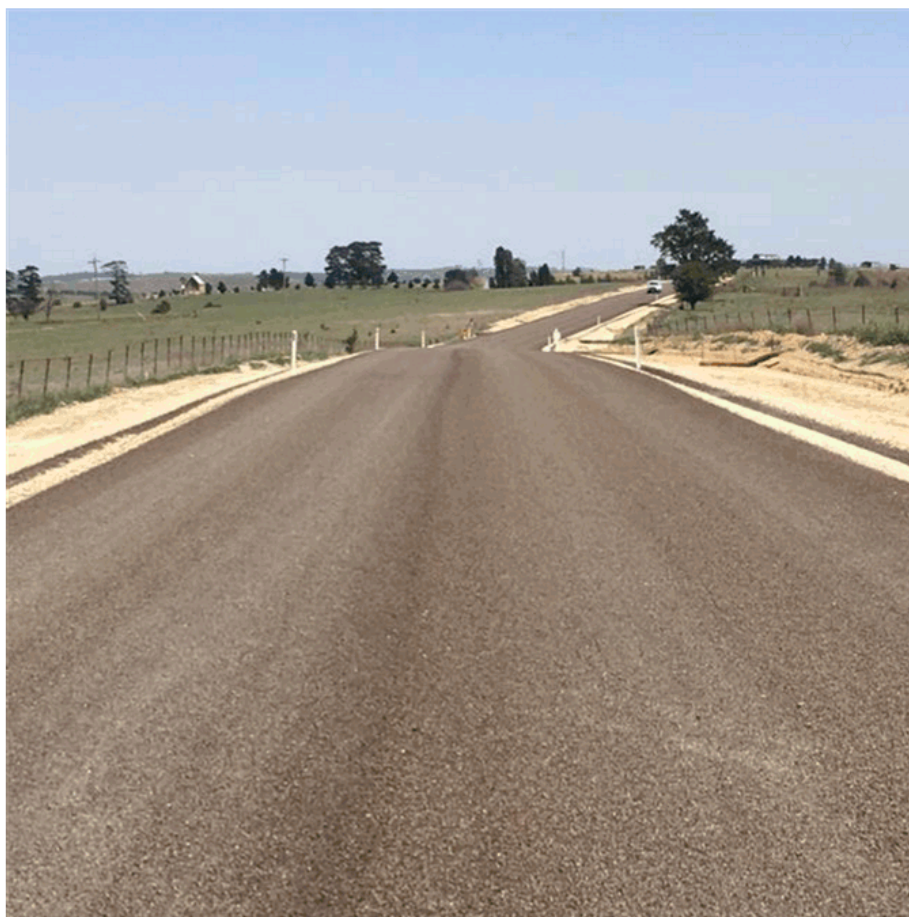
Gurrundah Road with final seal
