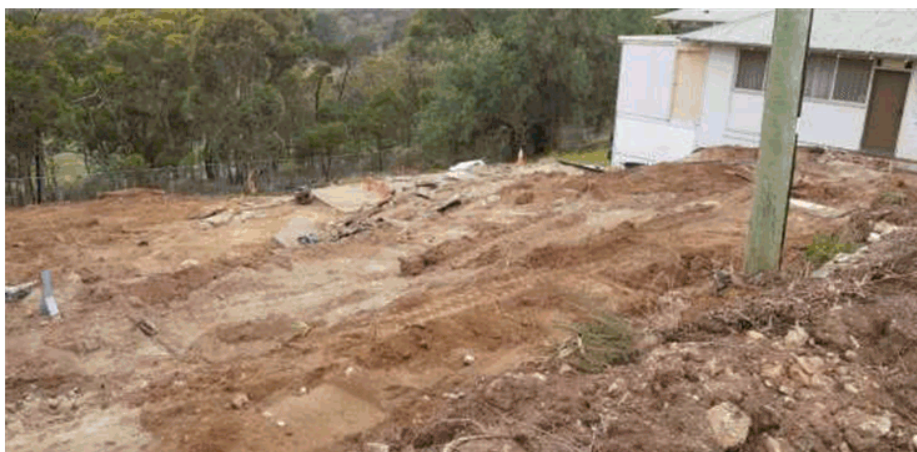
Above: works underway at Rocky Hill. Taken 1 February 2019
