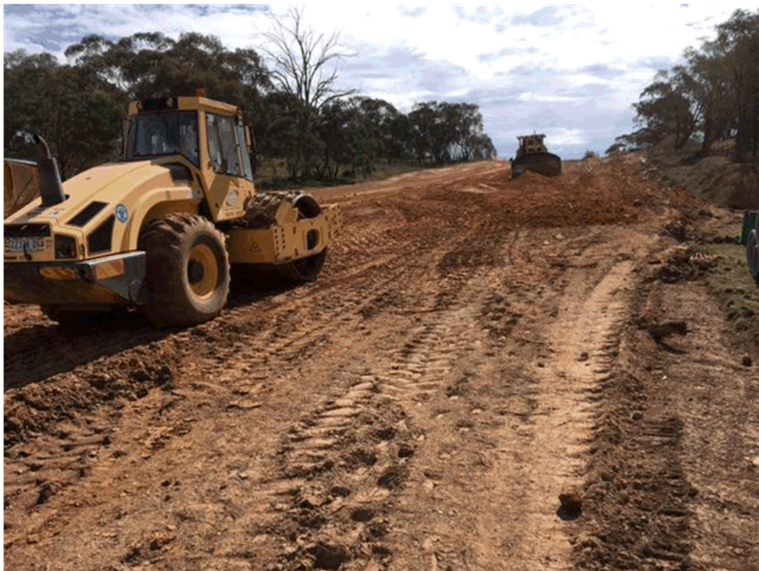
Mary Street Bulk Earth Works
