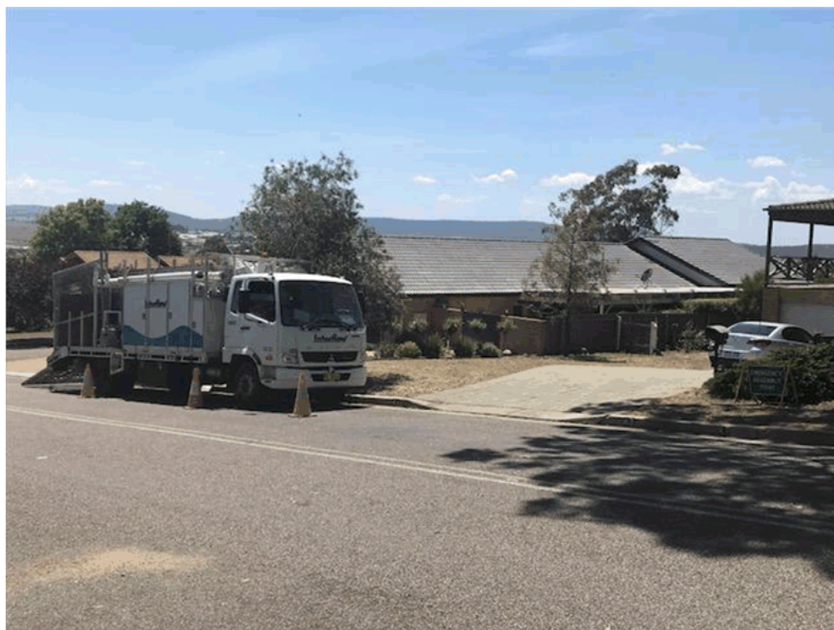
Interflow Relining crew
