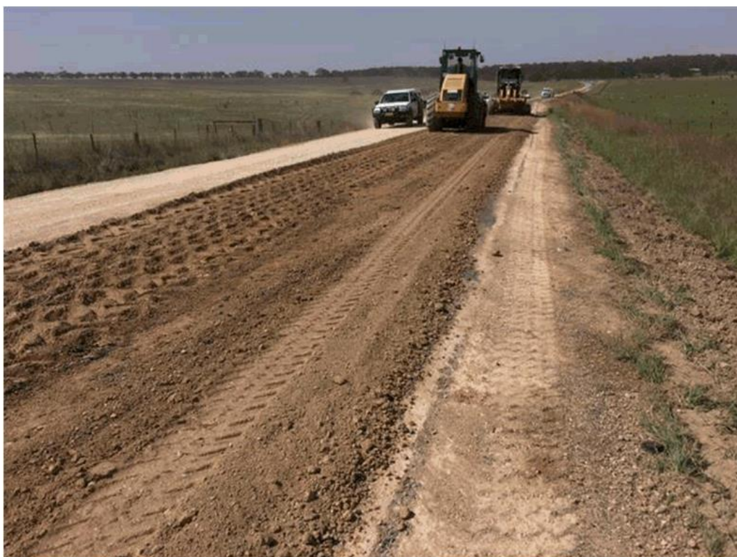
Windellama Road – Ripped ready for gravel overlay
