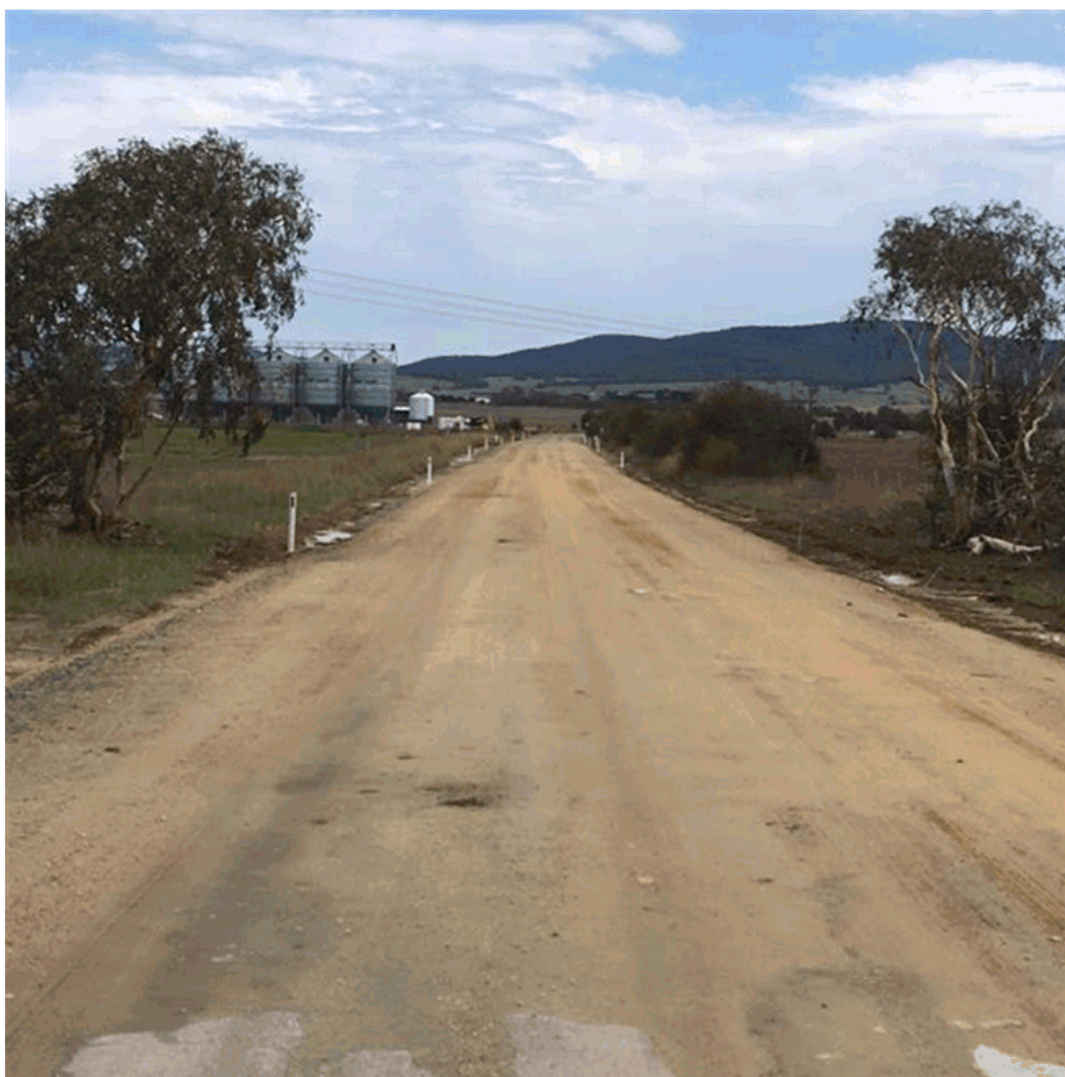
Currawang Road – Ripped and ready for gravel overlay
