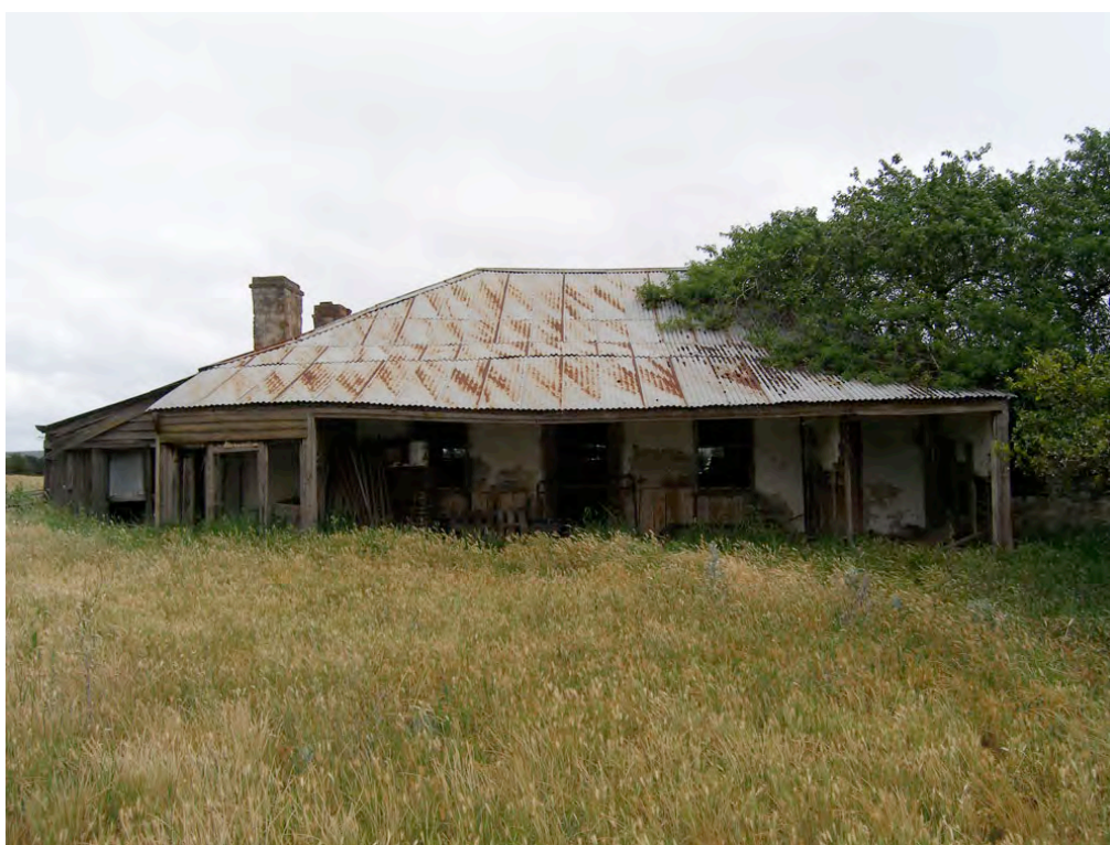
Inverary Park, Bungonia – The First Slab Cottage? – Edward Higginbotham 2009
