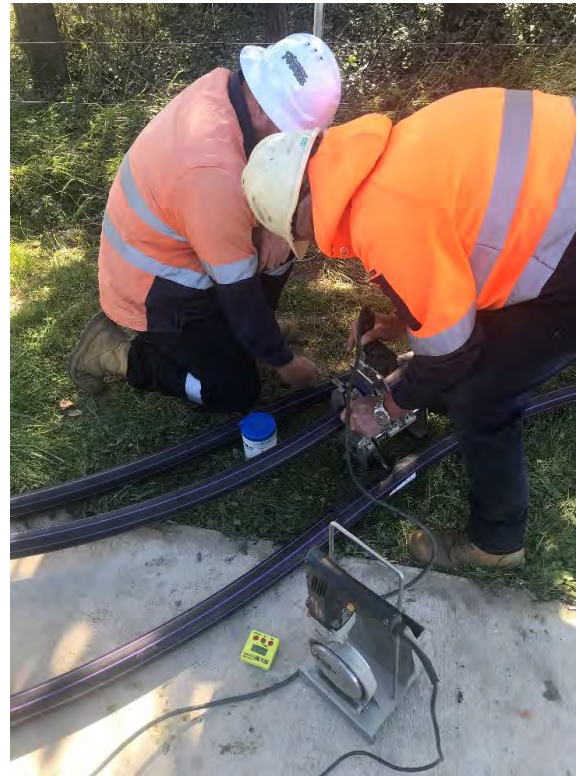
Bungonia Road Bridge Crossing
