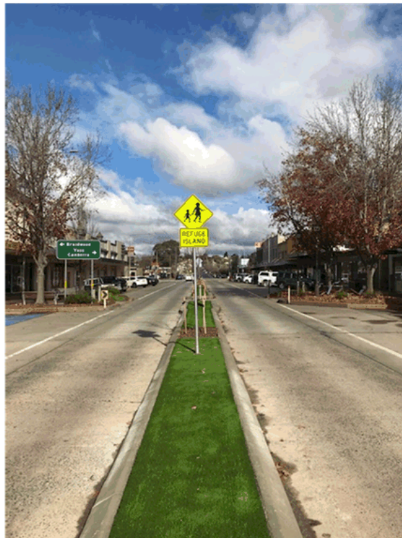
Auburn Median Replacement – Verner to Clinton Streets Synthetic Grass and Signs
