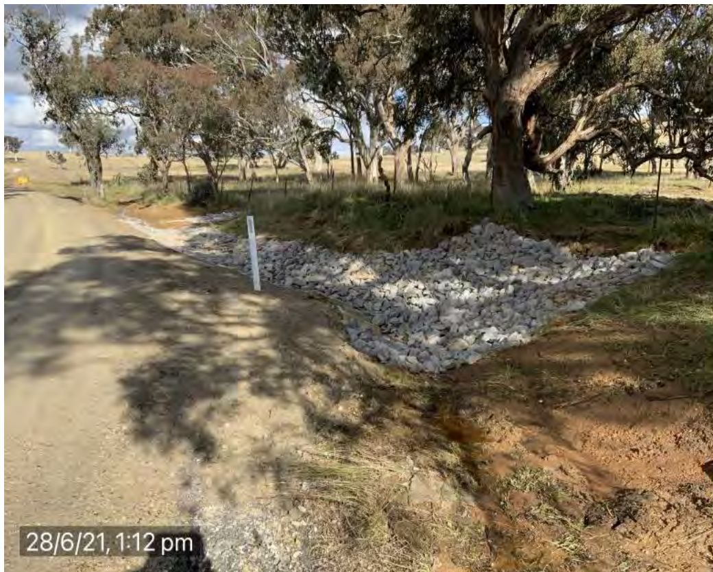
Erosion Repair works in progress on Wollogorang Rd
