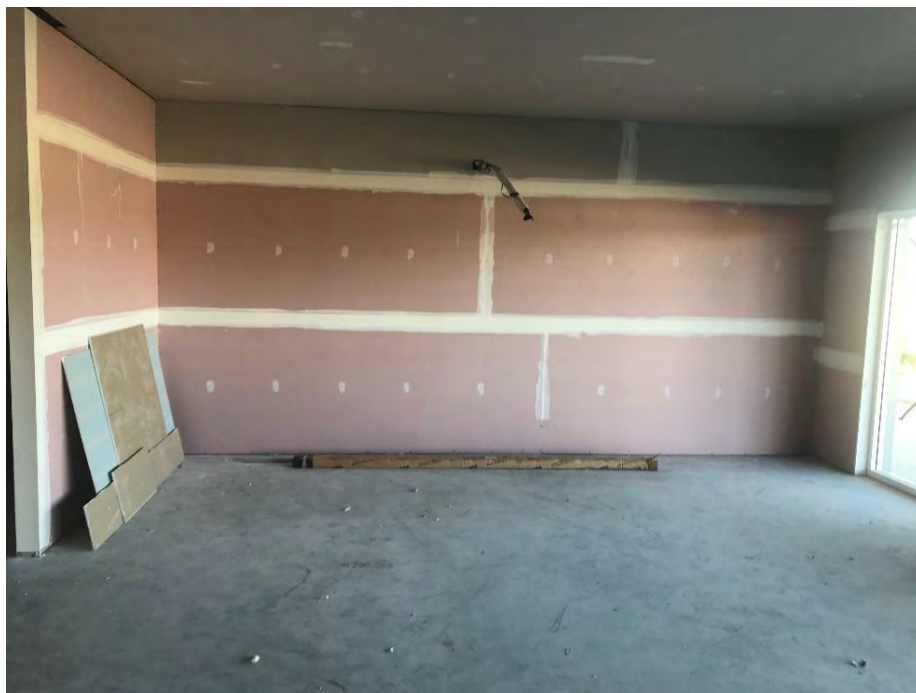
Cookbundoon Pavilion – Internal wall coverings (function room)
