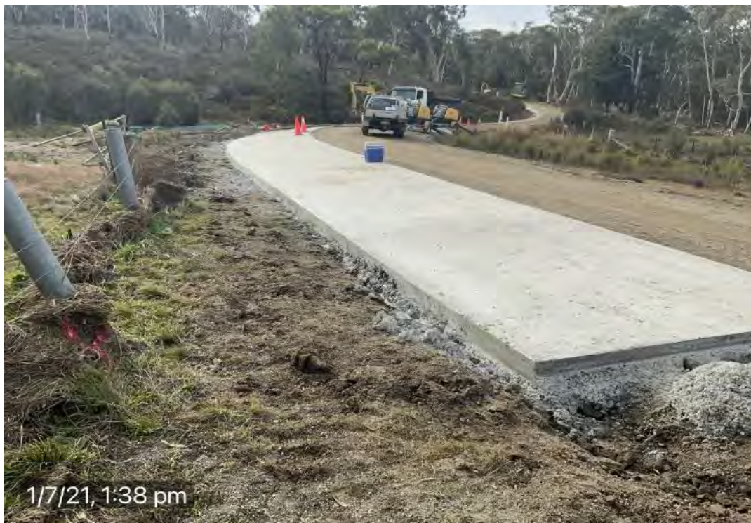
Causeway Erosion Repair works in progress on Barbour's Creek Road
