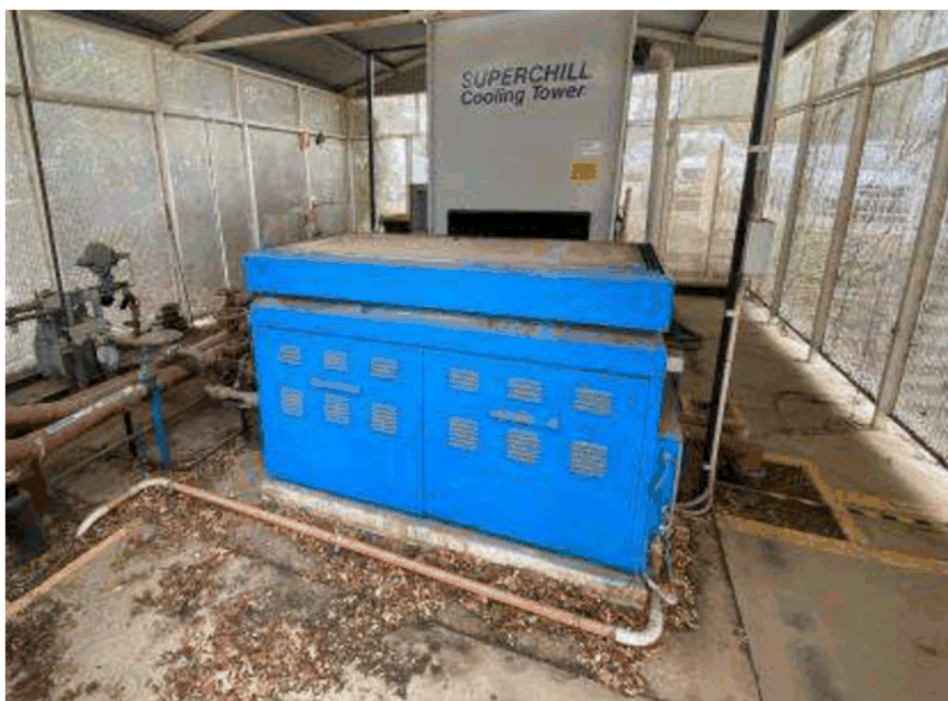
Main Boiler Civic Centre
