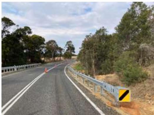
Guard Rail Installation- Stage 3 Works
