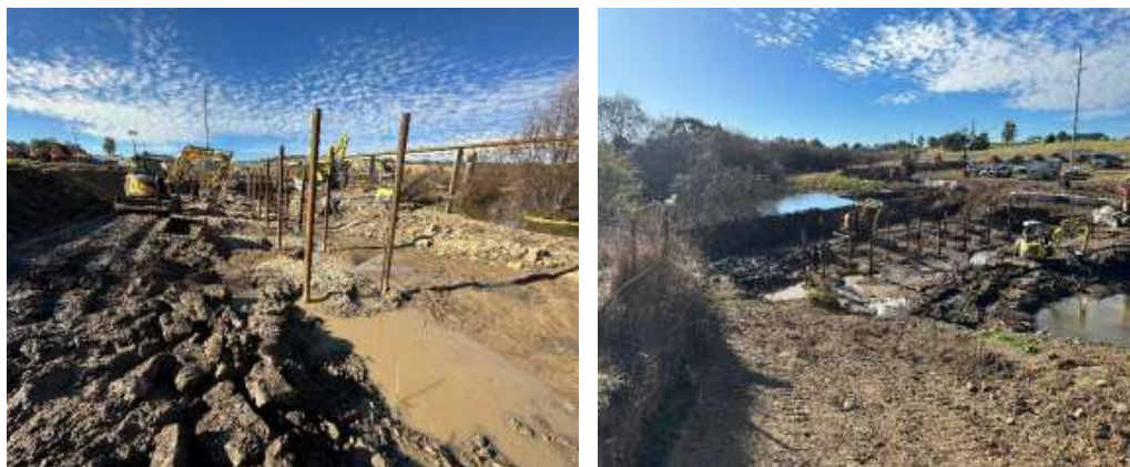
Wollondilly River Walking Track - Piling for river crossing
