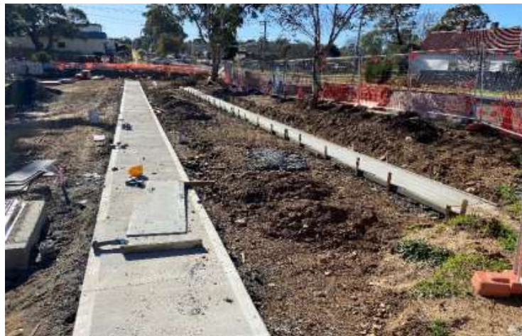
Faithfull Street Stormwater improvements
