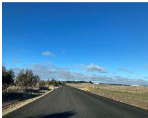
Bitumen Sealing Works – Stage 4 Section 2
