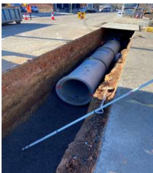
Bradley Street – Stormwater improvements
