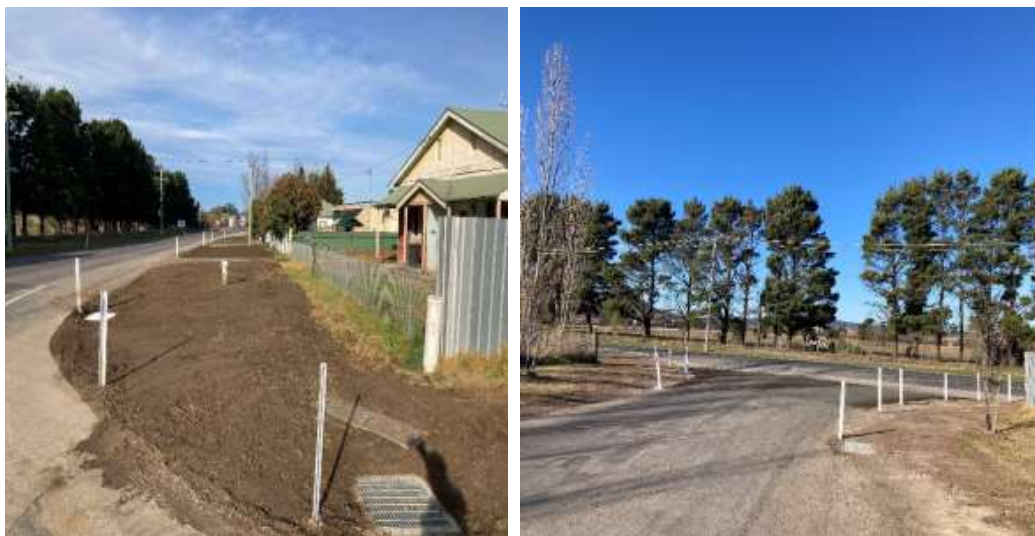
Garroorigang Street Drainage Work
