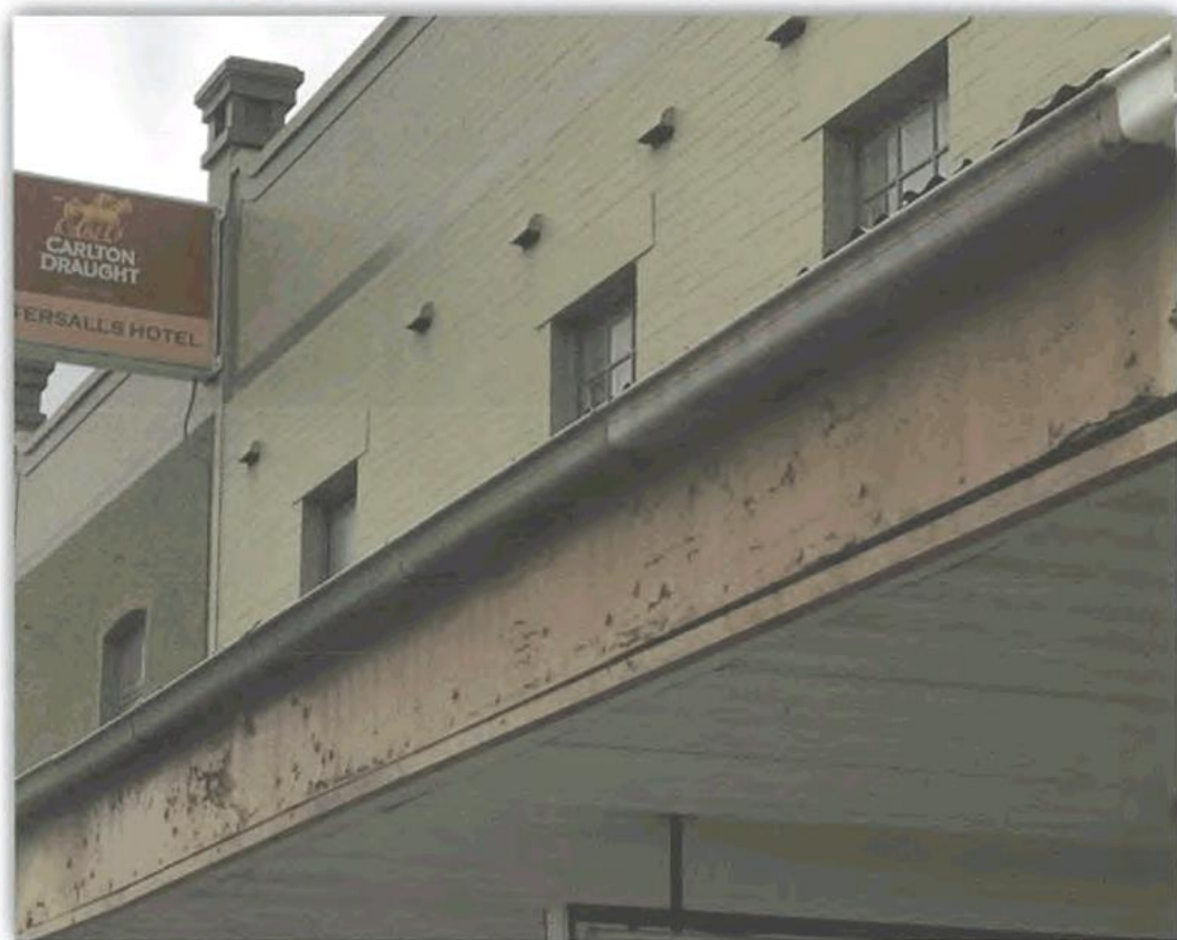
THE FACIA IS WEATHERED AND IN NEED OF REPLACEMENT AND PAINTING.
