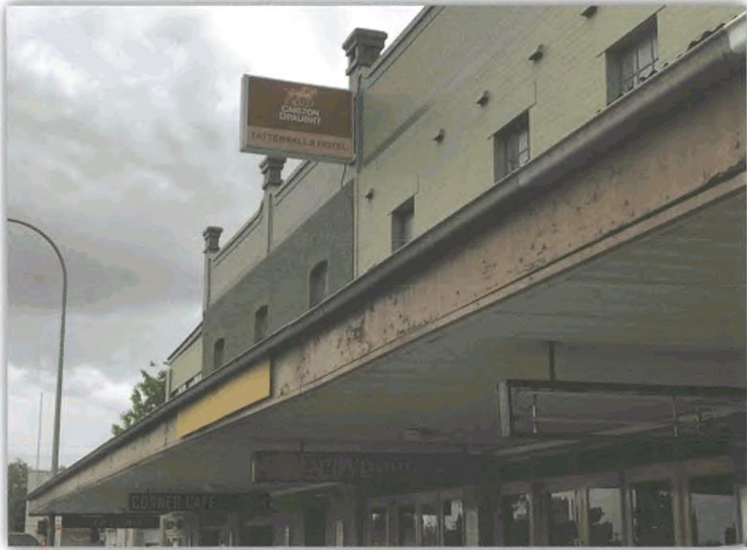
THE FACIA IS WEATHERED AND IN NEED OF REPLACEMENT AND PAINTING.
