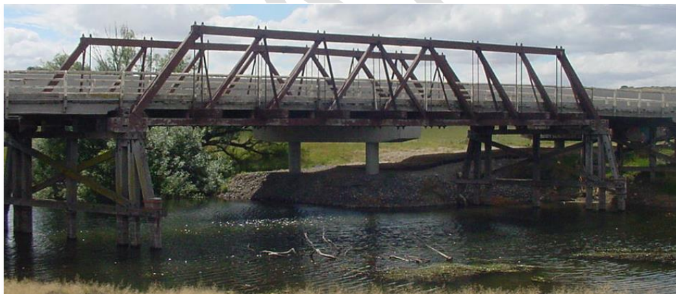
Photo: Mulwaree River Crossing, Braidwood Road.
