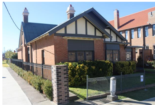
New Paintwork at 61 Verner Street, Goulburn
