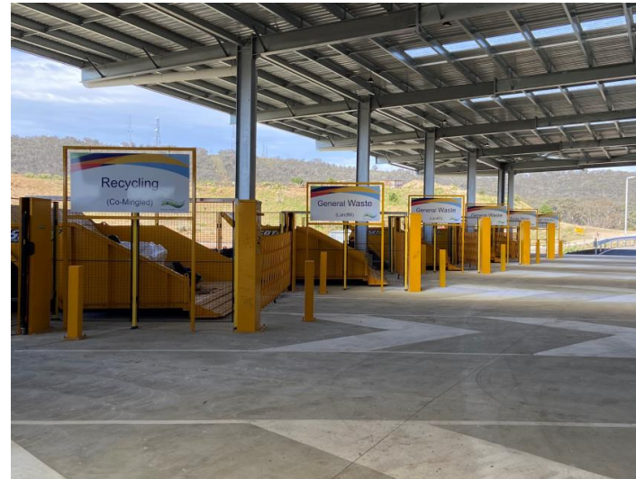
The newly completed Resource Recovery Centre disposal area
