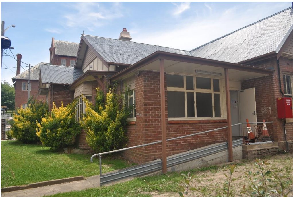
Three quarter view of the Southern elevation.
