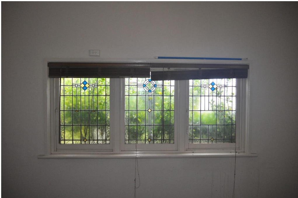
Existing original window – to be refurbished and retained
