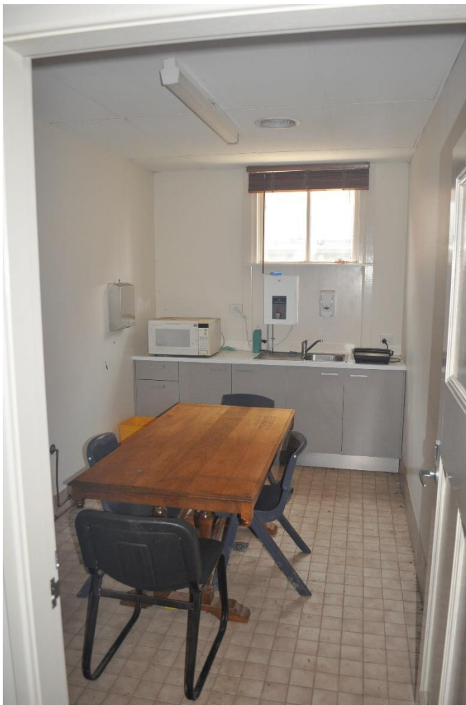
Small kitchenette conversion off the main hallway. The room will be stripped out complete and the full window reinstated
