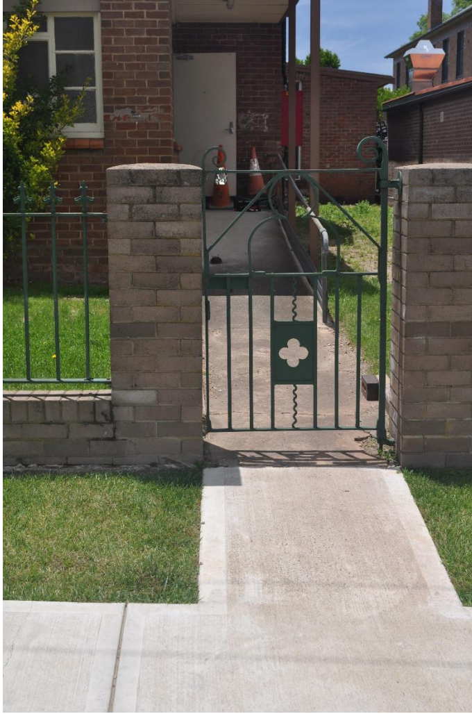
Detail of the existing front Gate.
