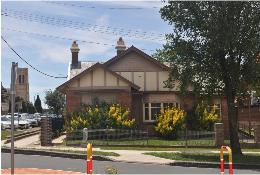
View of the Southern elevation. Note the St Saviors bell tower in the back left of frame
