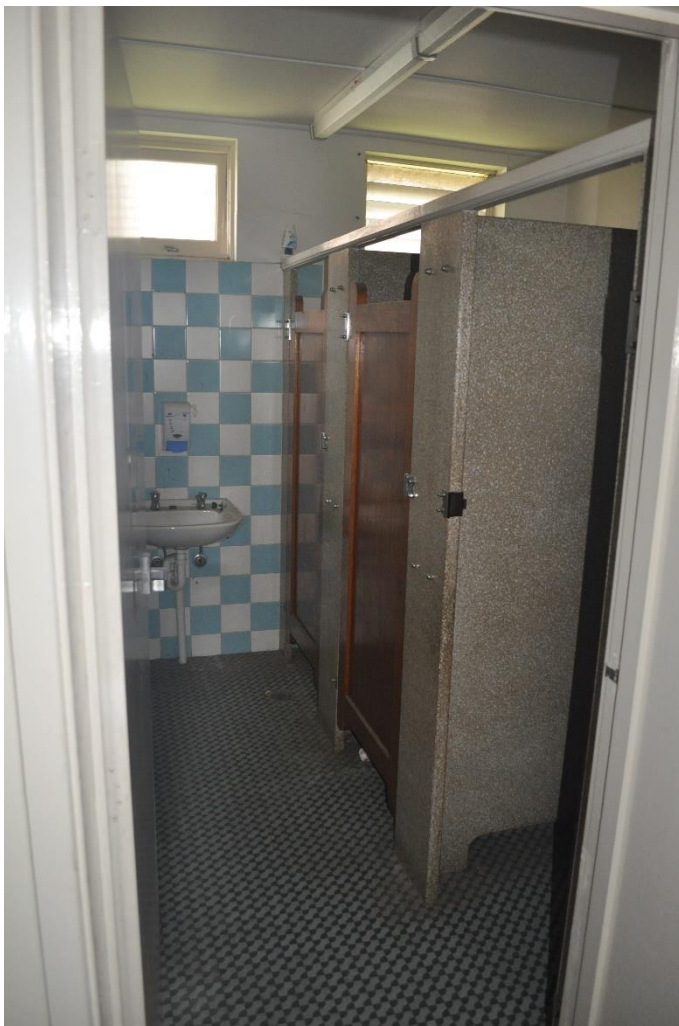
View into the female toilet section. To be stripped out complete.
