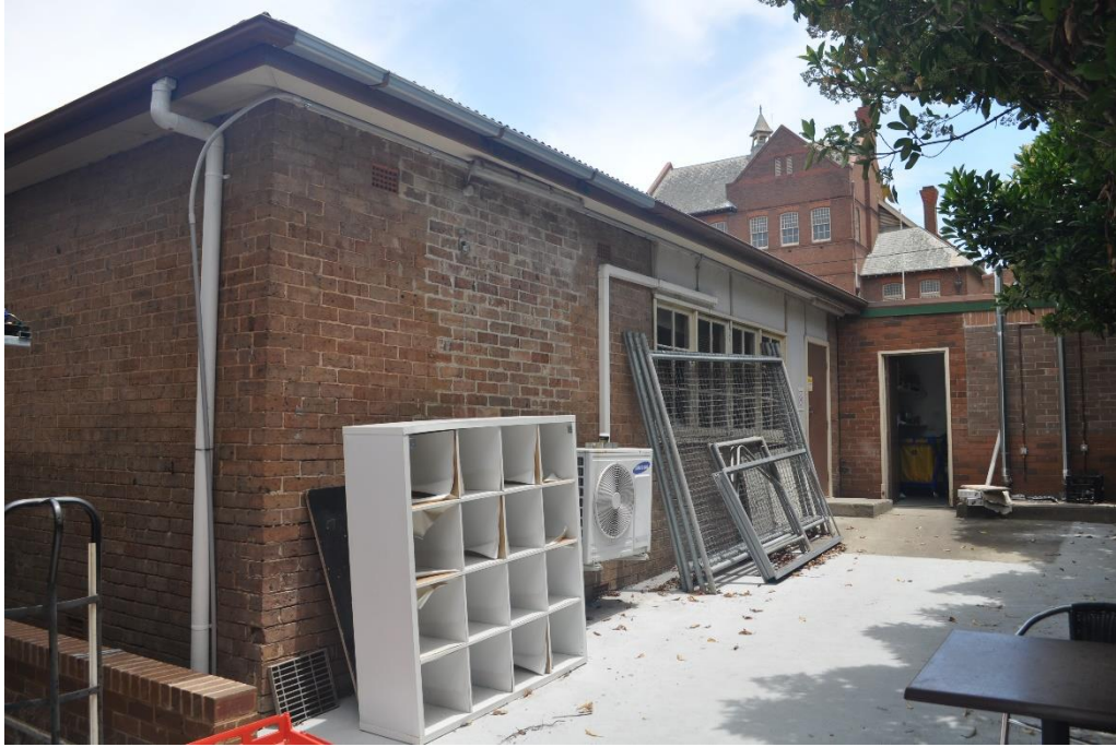
View of the north elevation
