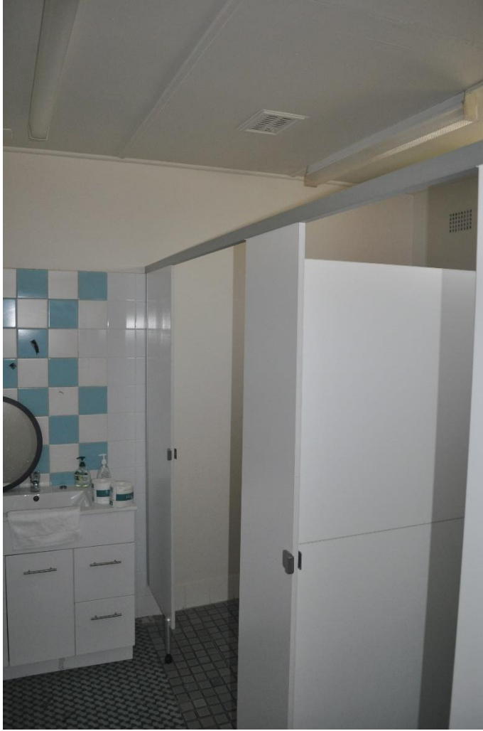
View of the existing accessible access
