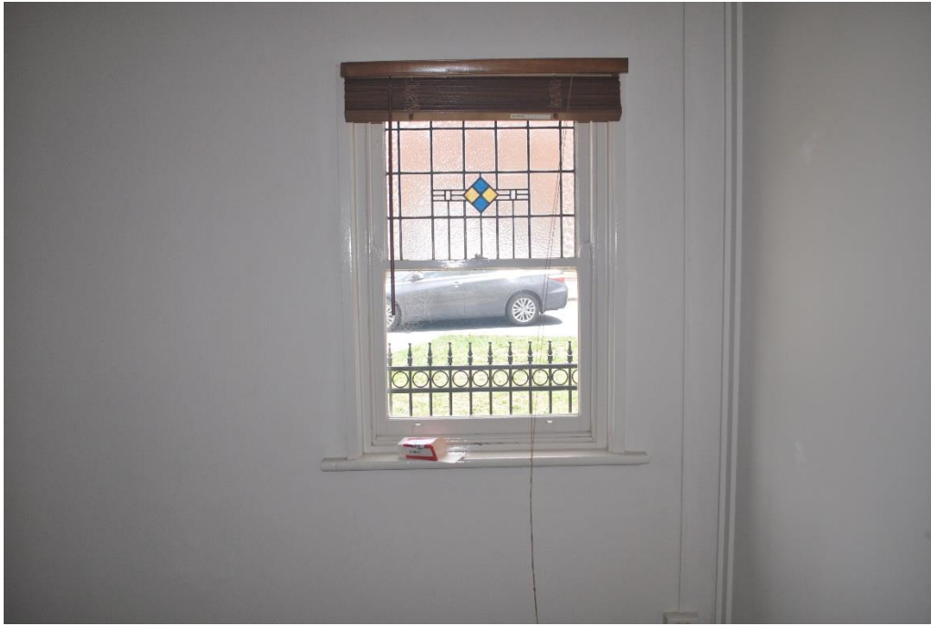
Original window facing Bourke Street (southwest front room)
