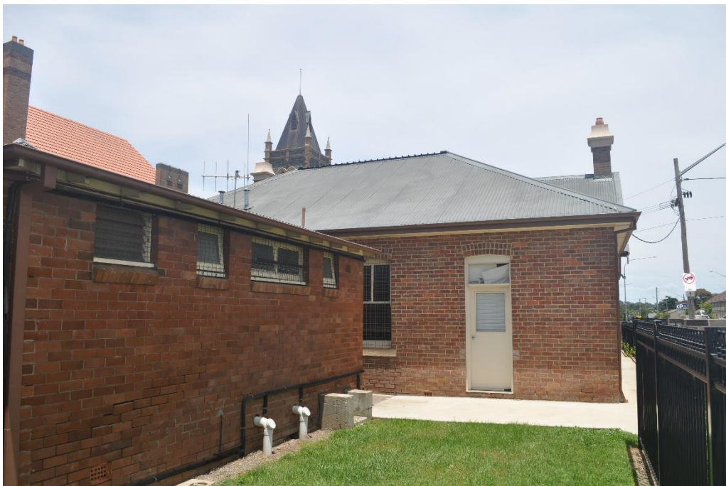
Partial northwest elevation. Note the access door. The proposed new work will remove the door and replace with a window into the proposed new accessible suite. The added ablution block is to the left of frame.
