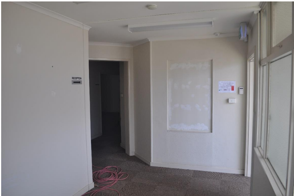
Internal view of the verandah looking toward the entry. The entry door will be moved and widened to meet code.
