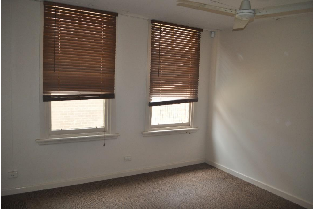
View of the North Eastern corner room of the original dwelling. Ceiling will be raised and the partition will be moved as per the new suite layout.
