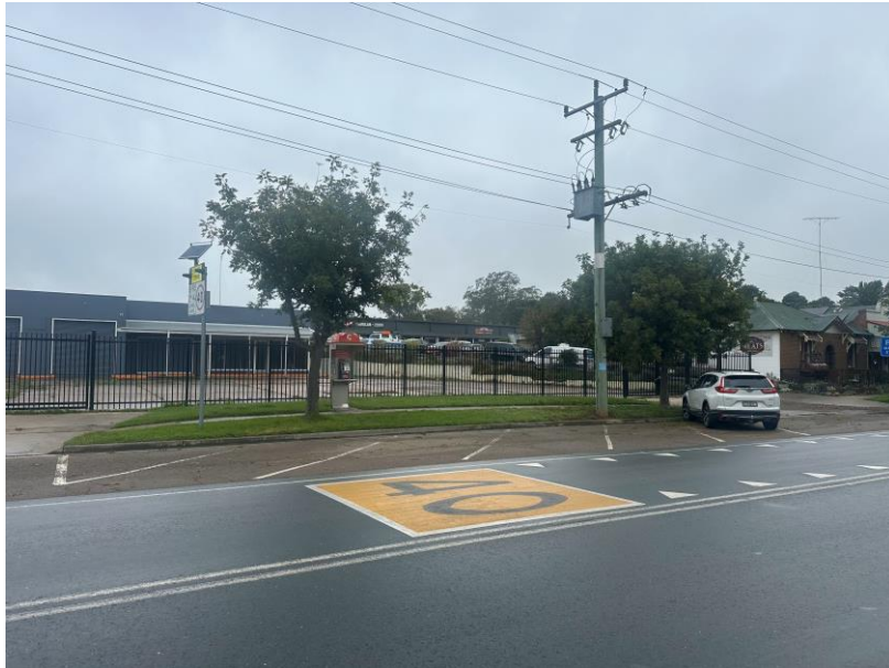
Figure 11: View looking southeast from George Street
