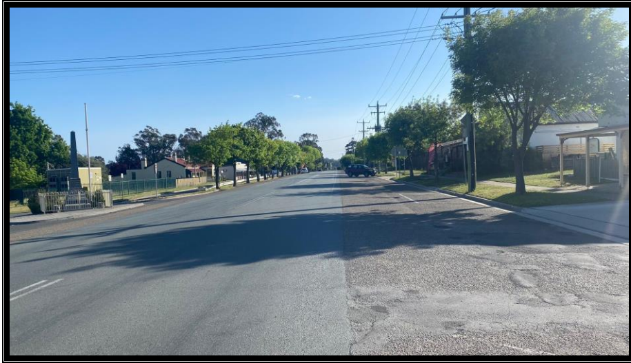
Photo 2: George Street at the subject site – facing north-east
