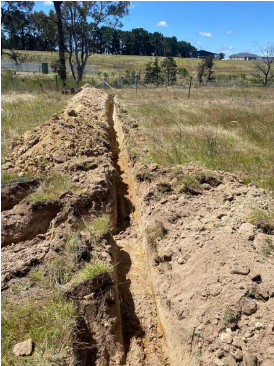
Figure 3: on-site Soil assessment.
