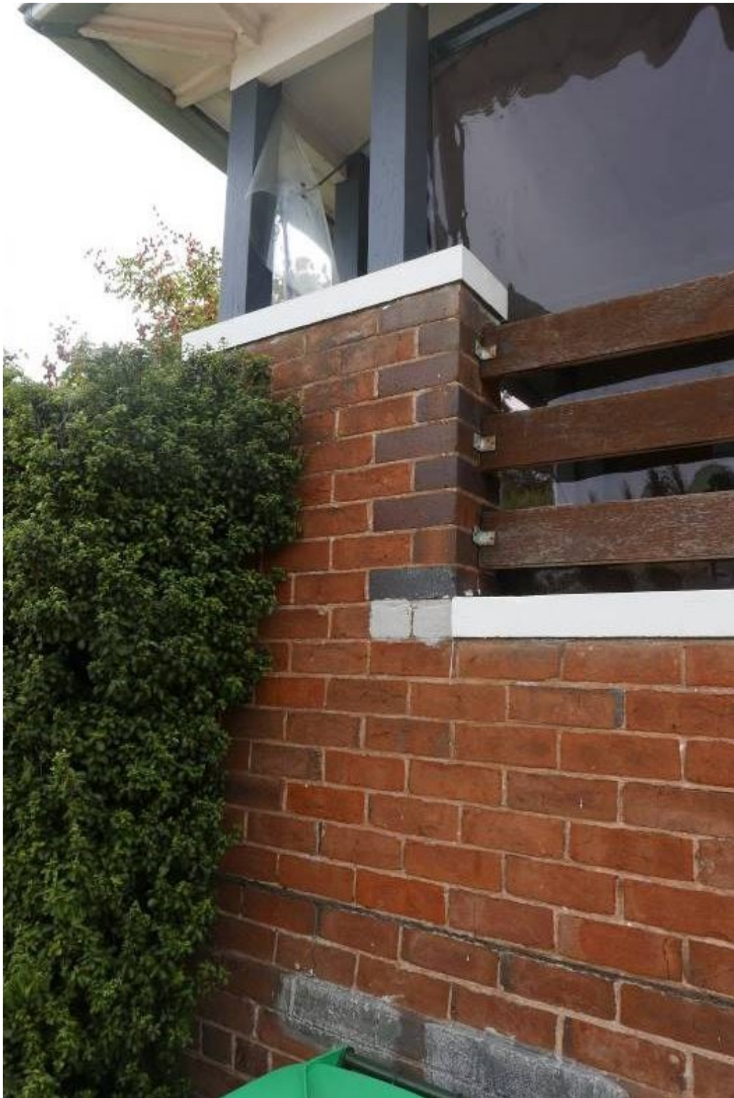
Photo 15 – Typical condition of porch wall capping.
