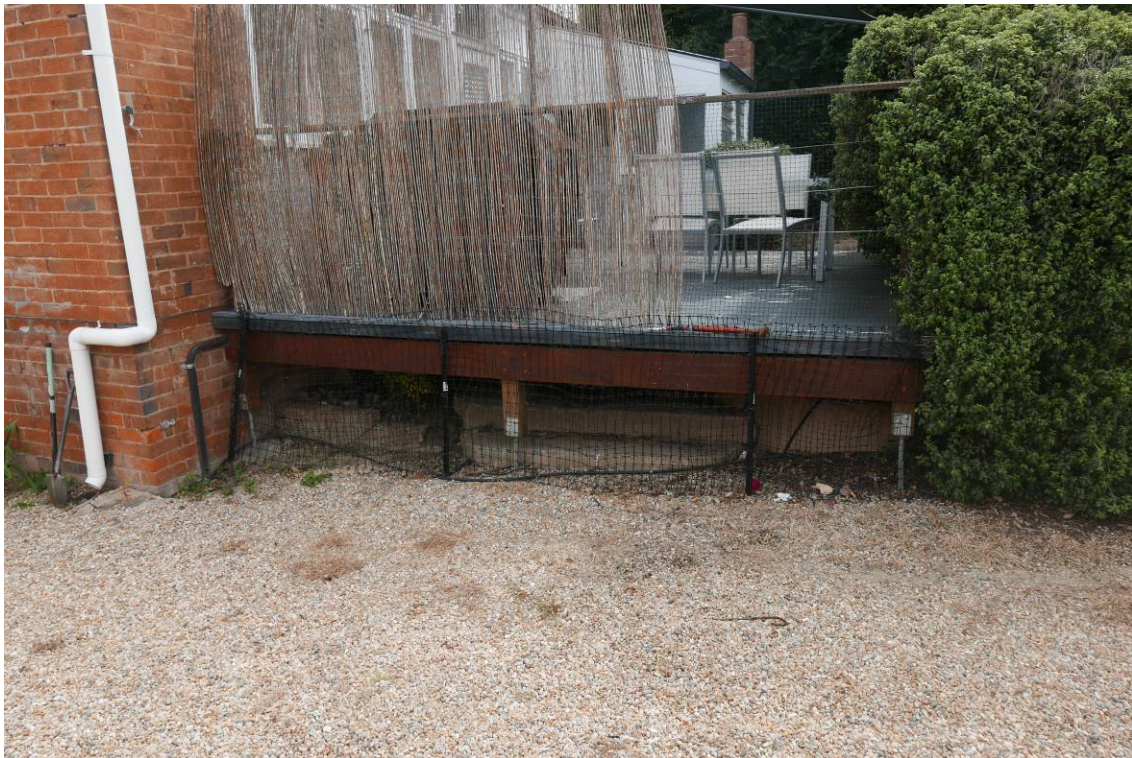
Photo 11 – Timber deck on the rear of the existing dwelling.
