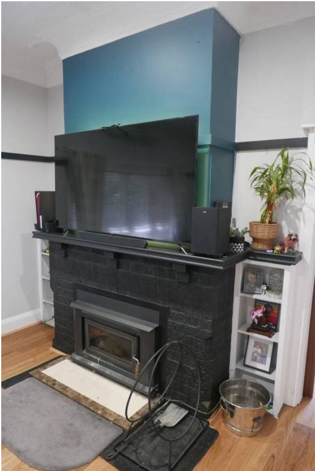
Photo 3 – Modified original fireplace in living room.
