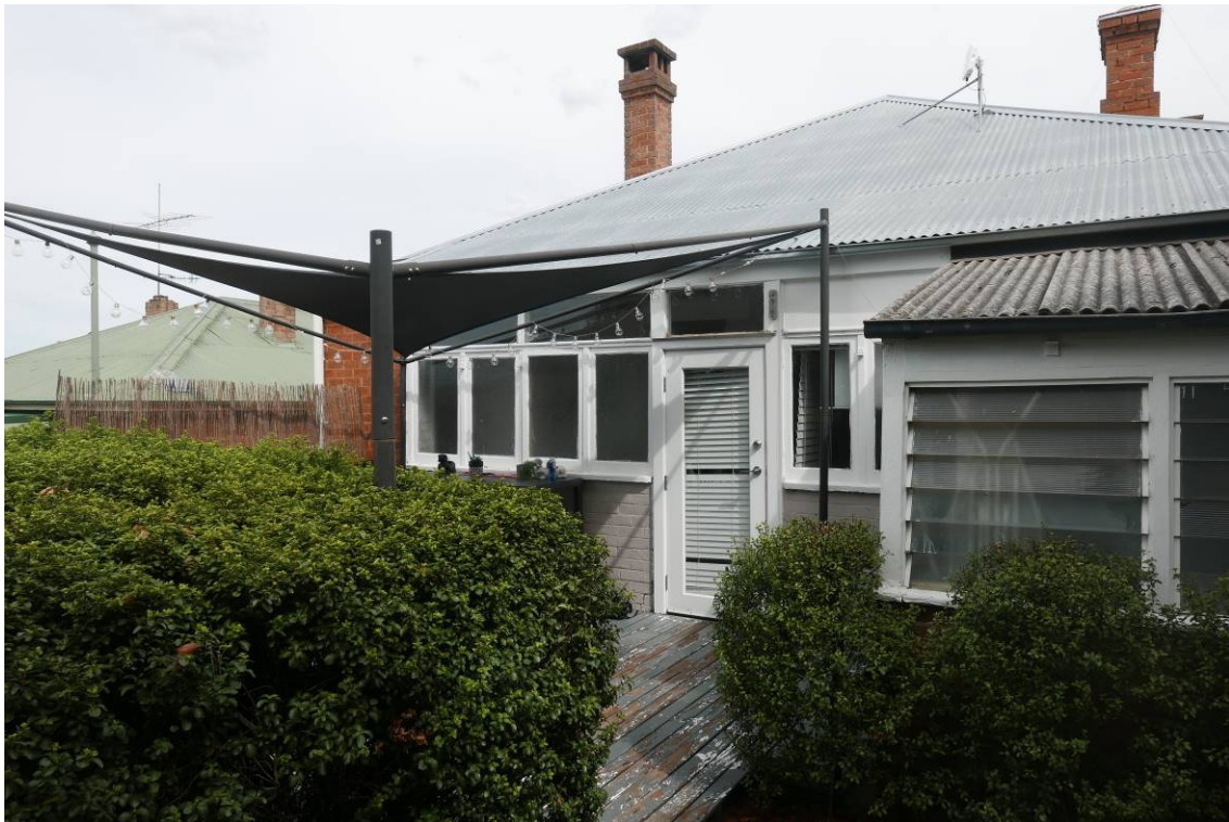
Photo 13 – Timber deck on the rear of the existing dwelling.
