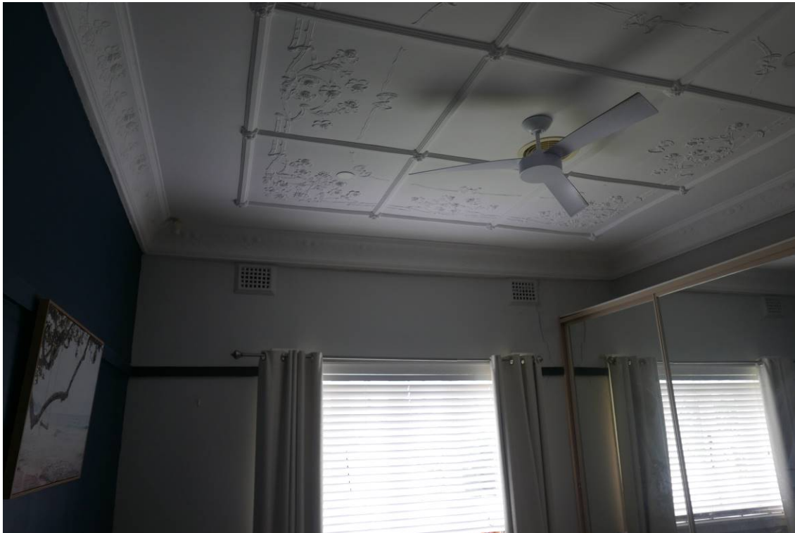
Photo 1 – Original decorative ceiling in front bedroom.
