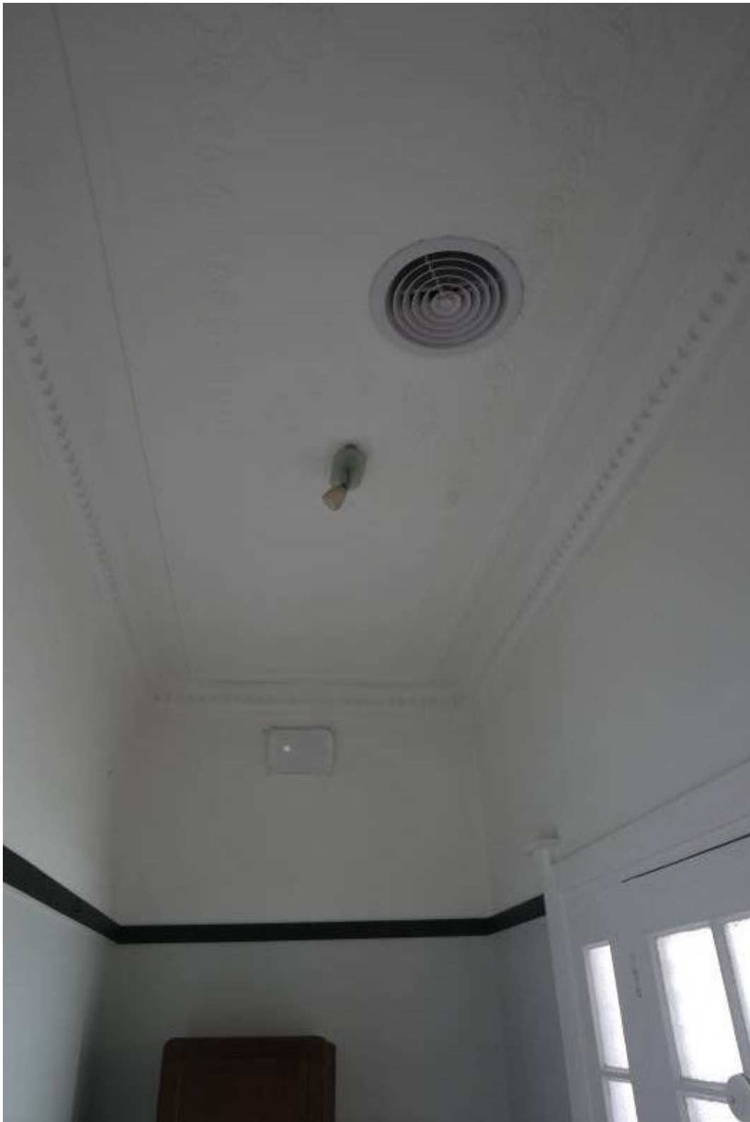
Photo 11 – Original decorative ceiling in entry foyer.
