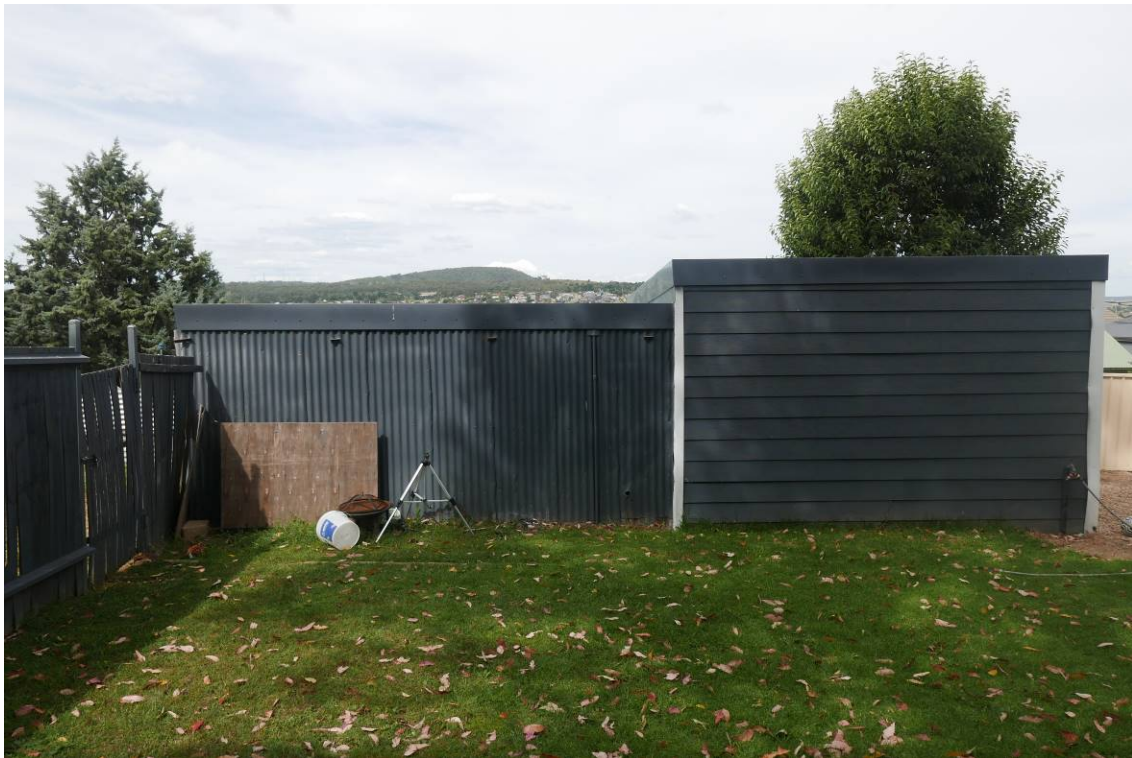
Photo 5 – View of existing shed.
