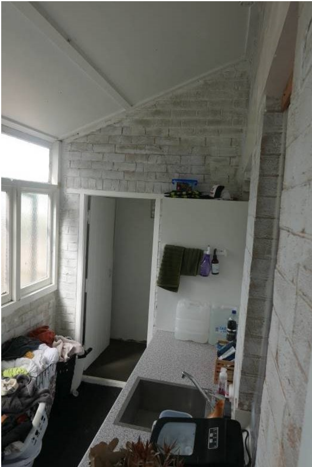
Photo 9 – Existing rear verandah enclosed. Laundry sink and joinery installed.
