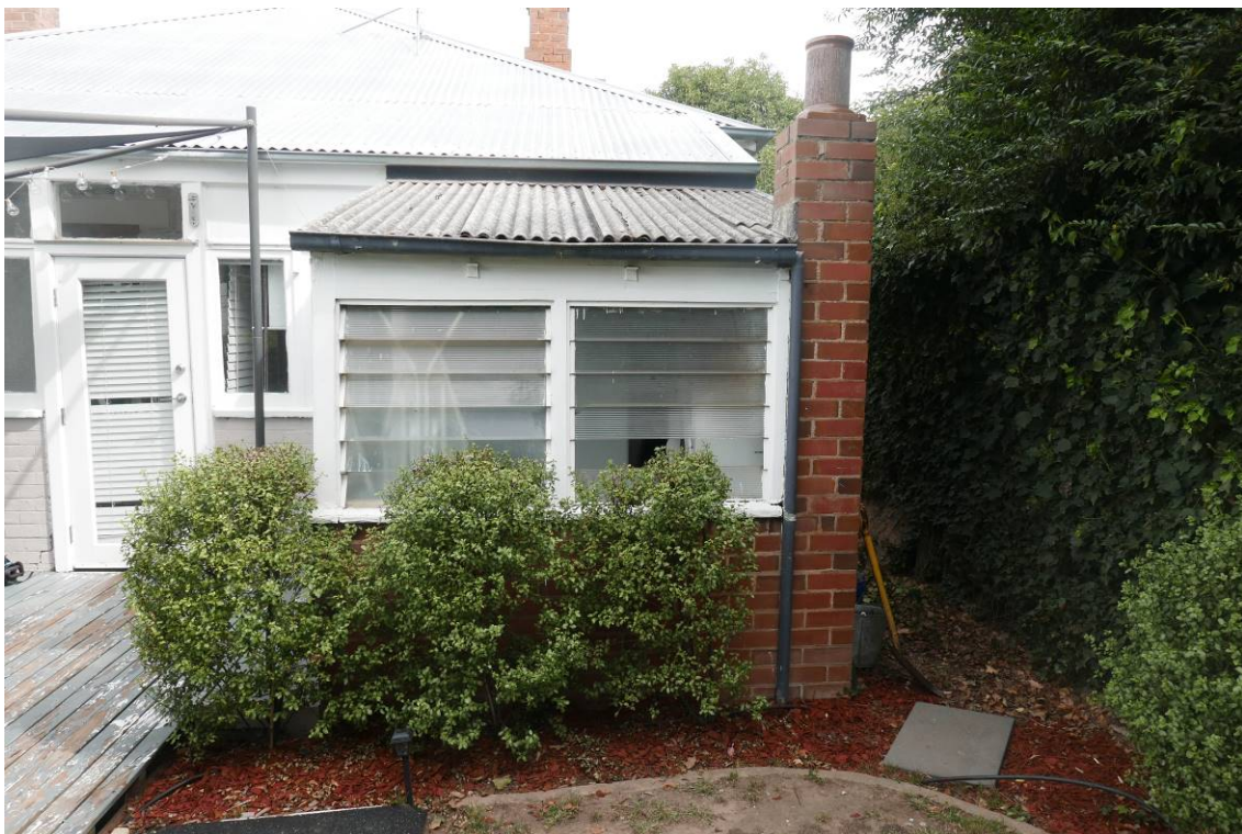
Photo 12 – Enclosed lean-to with brick chimney that houses the laundry.
