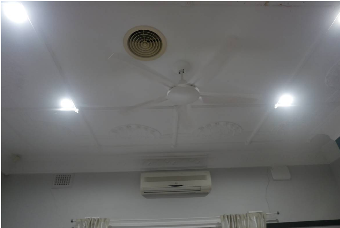
Photo 4 – Original decorative ceiling in living room.
