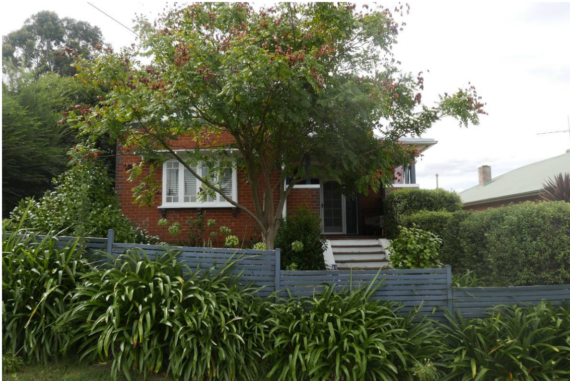
Photo 3 – Front view of existing dwelling.
