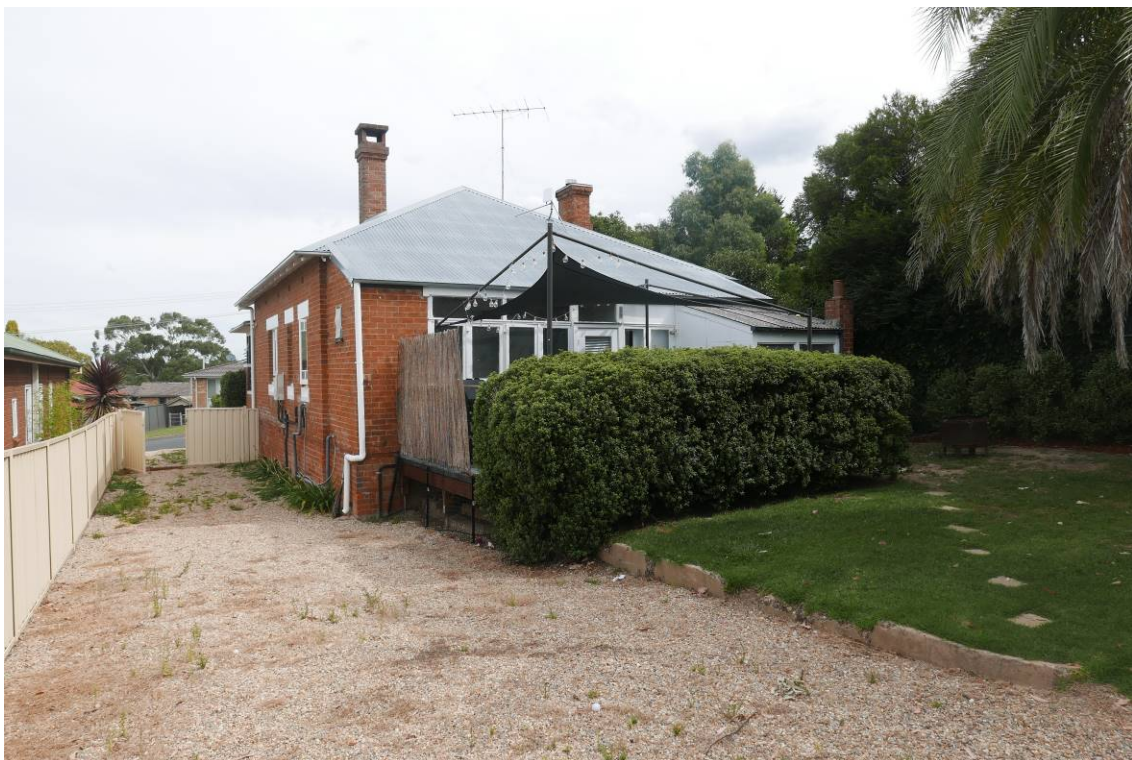
Photo 4 – Rear view of existing dwelling.
