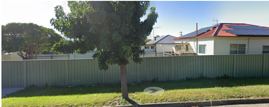
Dwelling from Furner Street
