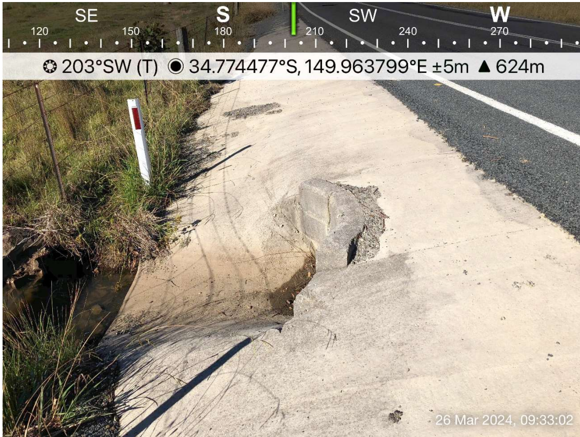
Existing pipe culvert to be upgraded to 600 mm diameter.
