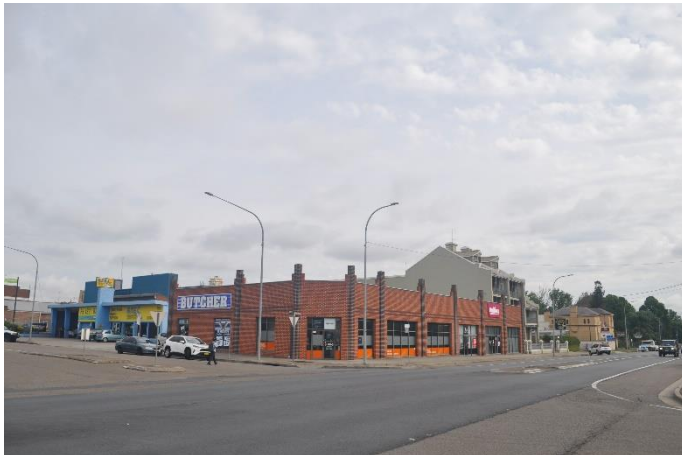
Figure 138 – Image Tim Lee Architects View of the site looking to the North toward Belmore Park along Sloane Street.
