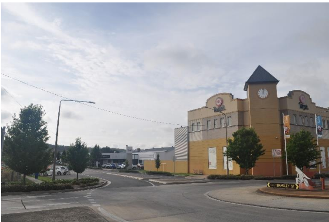
Figure 67 – Image Tim Lee Architects View of the site from the Bradley/ Auburn Street intersection
