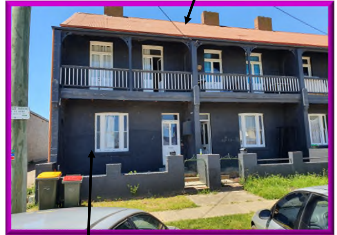
Grey painted facing brickwork
