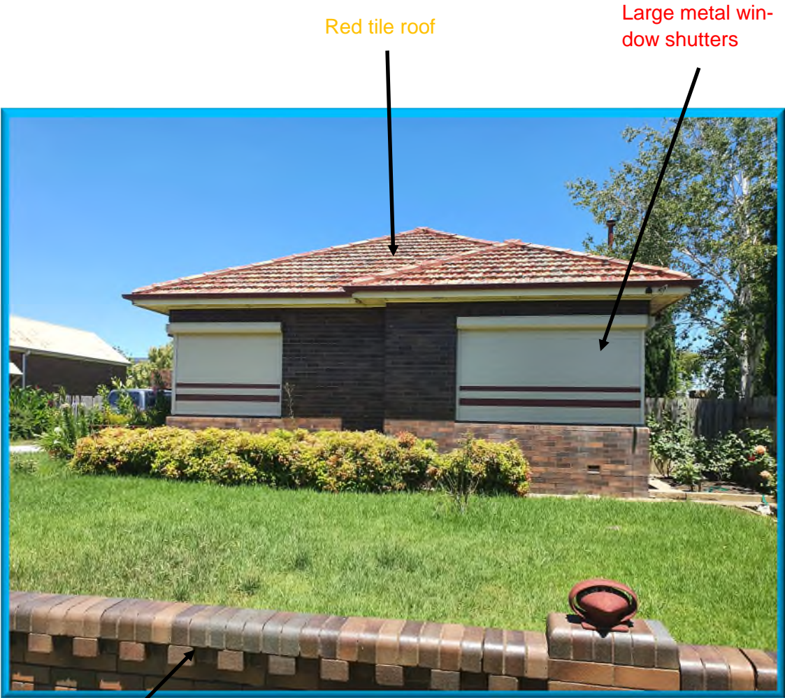
Low rise front brick wall with bullnose coping stones and corbelling detailing
