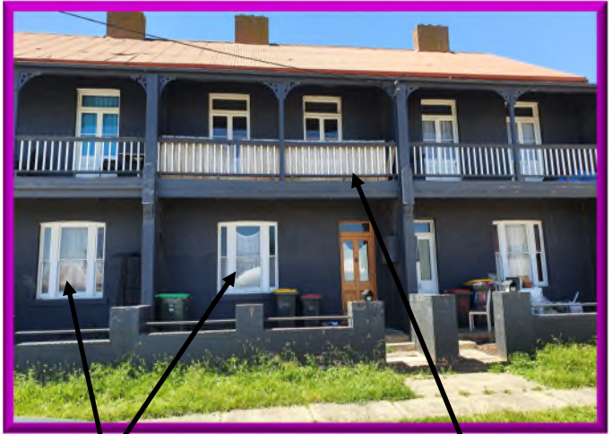
Timber double hung windows with side lights
