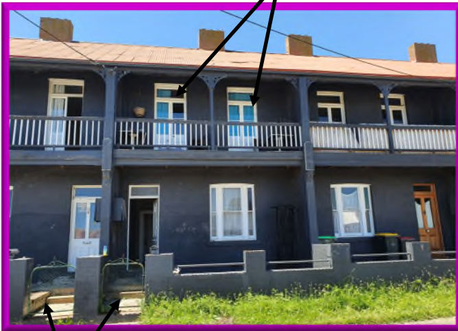
Wire mesh gates
