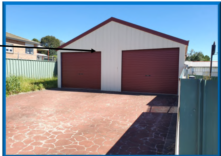
Cream painted timber weatherboarded façade
