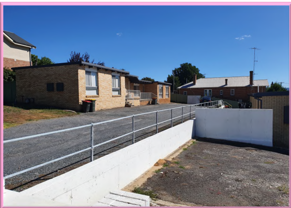
Large aluminum framed windows
