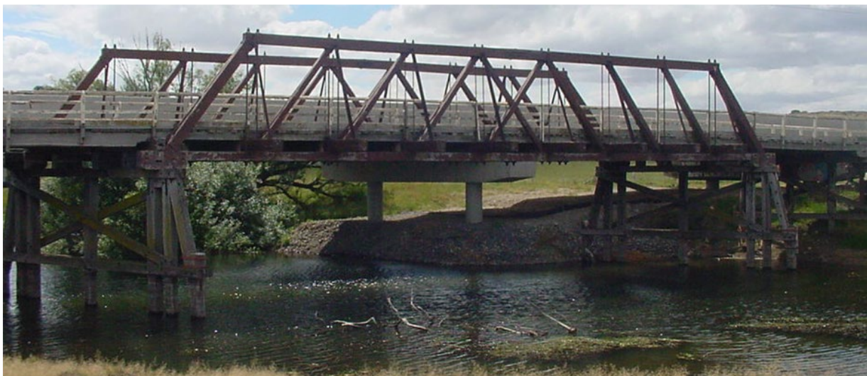
Photo: Mulwaree River Crossing, Braidwood Road.
