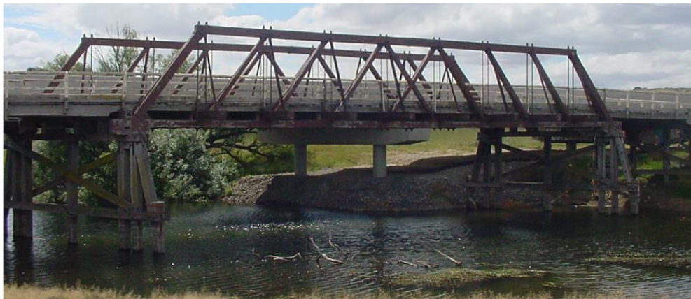
Photo: Mulwaree River Crossing, Braidwood Road.
