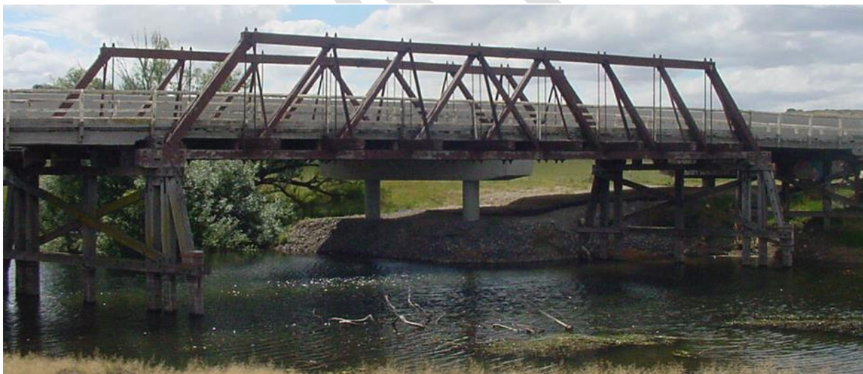
Photo: Mulwaree River Crossing, Braidwood Road.
