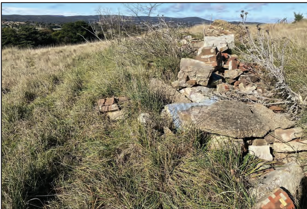
Photo 12: View of waste material on ground in fill platform area
