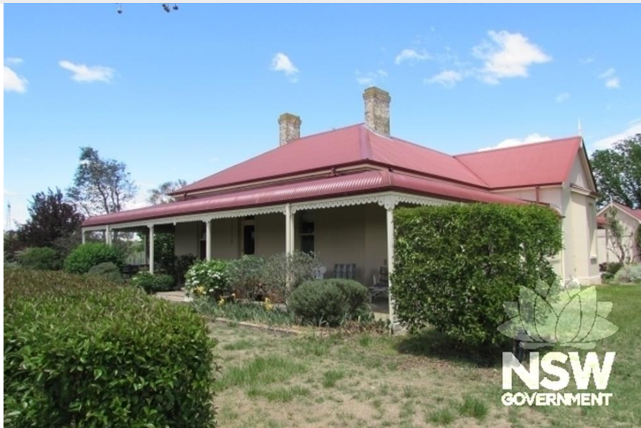
Local example 3- "Rosebank" 262 Windellama Road
